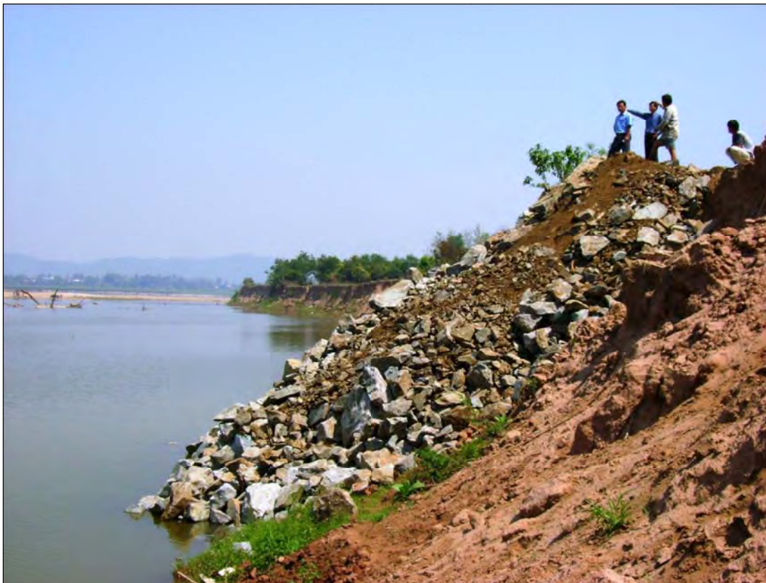
Figure 3-9 Hardpoint constructed along the Mekong for controlling river bank erosion.
