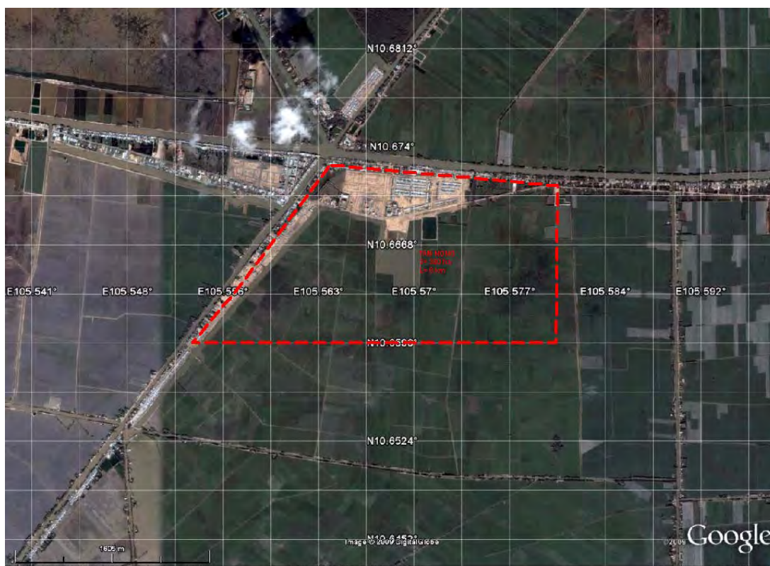
Figure 7-9 Flood control dyke in Tam Nong Town.
